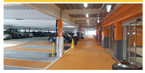
pedestrian walkways in a variety of colours including lilac and pastel orange. Overall, 10,500m2 of car parking was prepared, primed, embedded and coated in a high performance wear and waterproof membrane coating, while an additional 3,000m2 was prepared, primed and applied with Wearing Course on internal walkways. Ease of product application contributed to meeting the project's deadlines over a four-month period, with the first phase on levels three and four taking six weeks.
