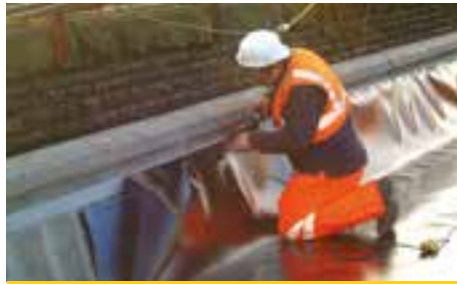
MONARD VIADUCT, CORK, IRELAND
